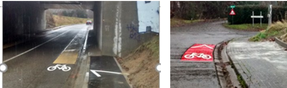
Figure 40: cycle path arranged over 100m with unsafe cycle path ending © Transport & Mobility Leuven
