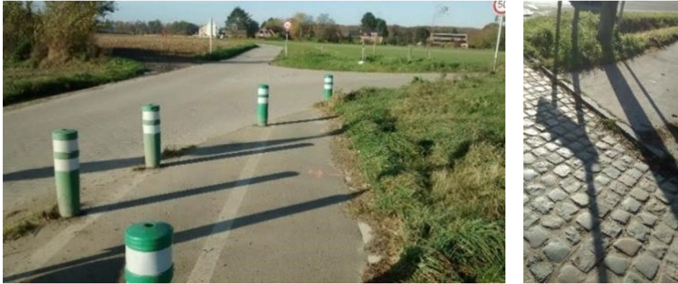
Figure 38 (left): unsafe start/end of a bidirectional cycle path at a crossing © Transport & Mobility Leuven.
