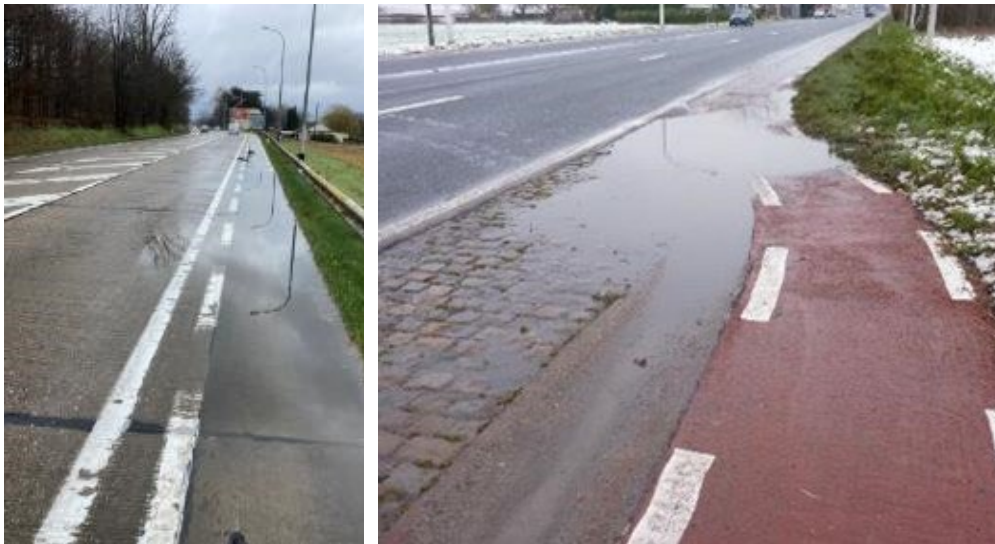
Figure 45: cycle paths with lot of water during and after rain making cycling very uncomfortable © Transport & Mobility Leuven.
