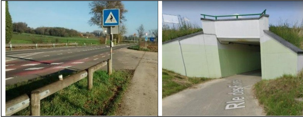
Figure 37: crossing of a heavily used road with 90 km speed limit, left an unsecure crossing with only some markings, right a cycle tunnel under the same road © Transport & Mobility Leuven.
