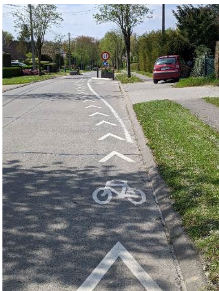
Figure 15: illustration of how the markings guide the trajectory a cyclist should follow to limit danger of getting squeezed between car and obstacle ©Transport & Mobility Leuven.
