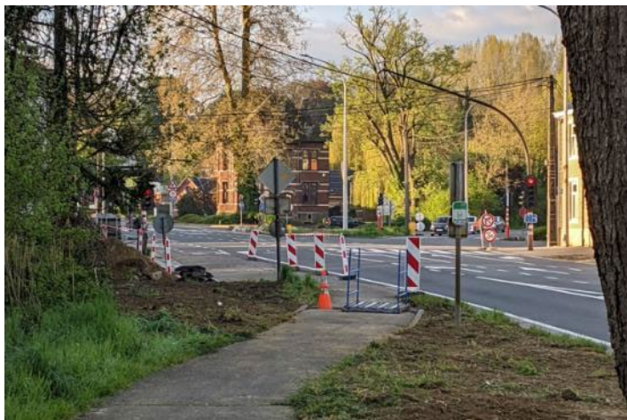
Figure 47: uncomfortable crossing during works at the cycle path © Transport & Mobility Leuven
