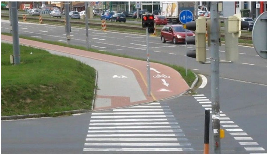
Figure 42: bi-directional cycle path in Ostrava, Czech Republic. © Mark Wagenbuur, bicycle Dutch, https://bicycledutch.files.wordpress.com/2012/08/ostrava.jpg .
